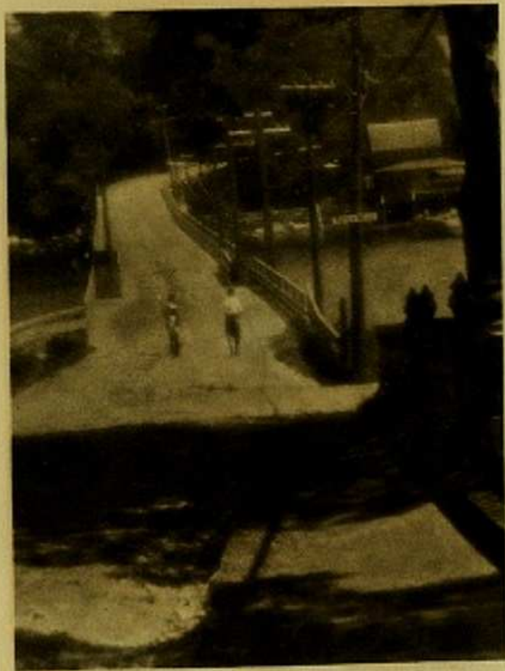
ARTHUR HAMMOND SUNLIGHT (AMERQUAN BRIDGE) BOSTON, MASS.
